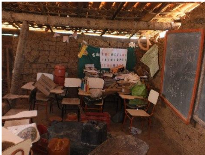
Image 1 – Rural public school in the municipality Xiquexique - BA. Source: https://avozone.com/2013/02/a-realidade-do-pessimo-estado-da.html
