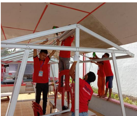
Figure 5. Aquaponic Instalation Framing in Detention Centre Dumai
