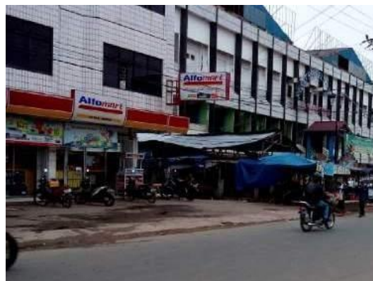
Figure 1. Violation of Minimarket Establishment in Hayam Wuruk Street.
