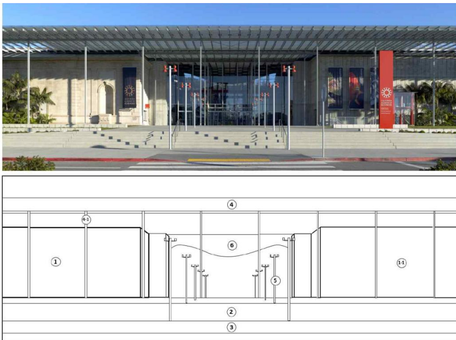
Figure 3. Facade Elements of the Front Entrance
